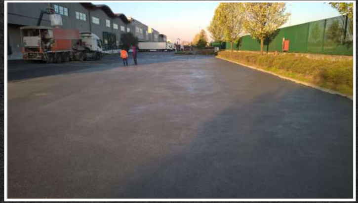
View of new applied asphalt
